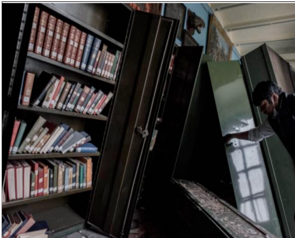
Figure 2 . Kaiser Library in Kathmandu after the earthquake (Cozens, 2018)
