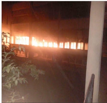
Figure 7. The Naraguta Campus library on library fire during the disaster (Sadiq, 2016)
