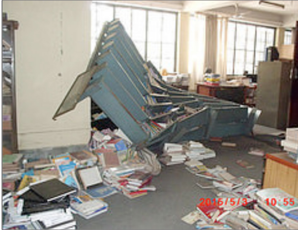
Figure 1 1 . Tribhuvan University Central Library after the disaster (“Nepal Library”, 2018)
